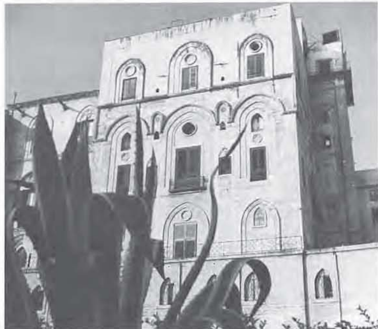
Palazzo dei Normanni, Palermo, Sicily. Built by the Saracens, enlarged by the Normans, and often altered, today it is the seat of Parlamento della Regione Siciliana. ICI
