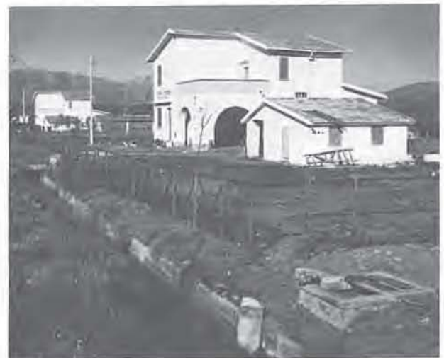
Lazio. Land reclamation in the south. Part of the Italian land reform program. EPA
