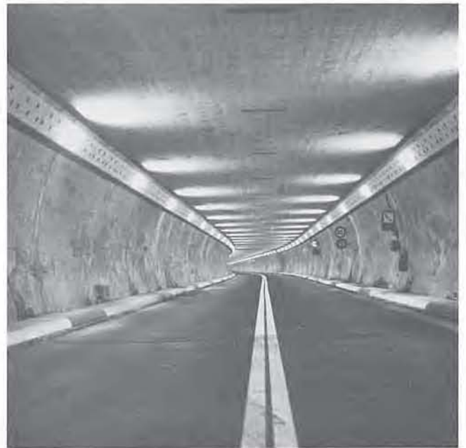
Tunnel through the Great Saint Bernard Pass between Martigny-Ville, Switzerland, and Aosta, Piedmont. EPA
