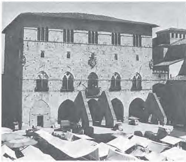
Palazzo del Comune, Pistoia, Tuscany. A massive sandstone structure built by the Guelphs in 1294, and later enlarged. EPA
