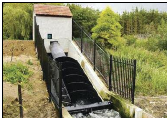
A working Archimedes' Screw in Holland.
