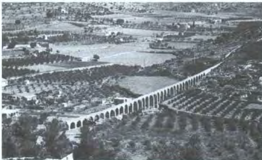
A Roman aqueduct crossing the Spanish countryside.
