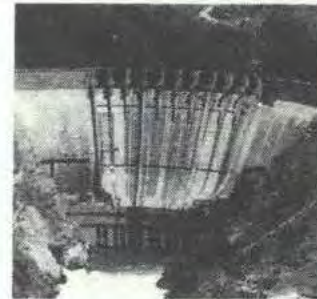
Hydro Plant in Turkey
