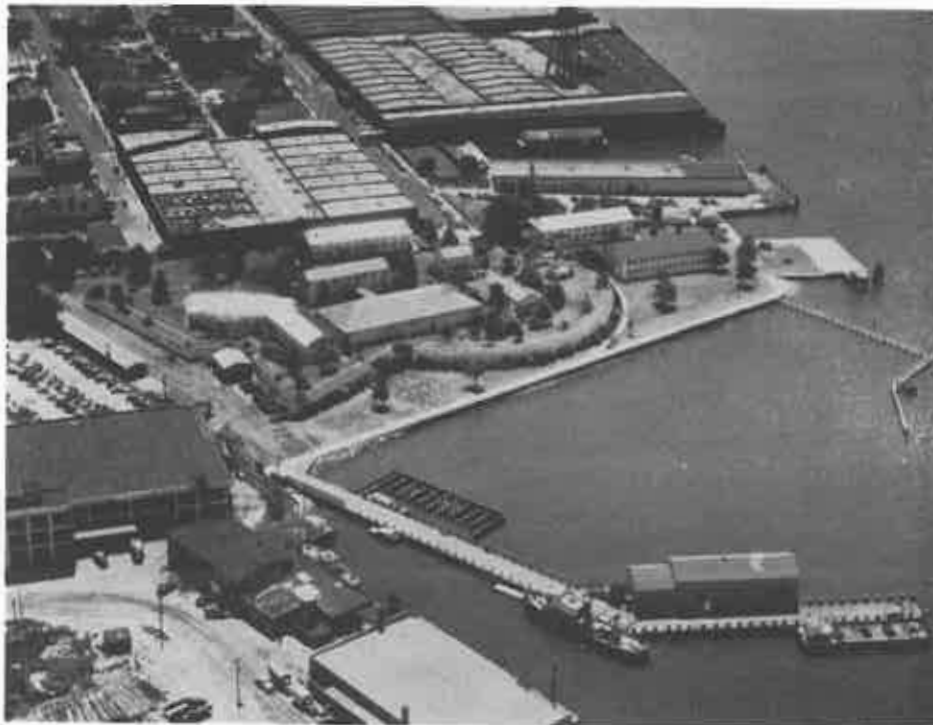
AIR VIEW OF FORT NORFOLK TODAY (Courtesy, Corps of Engineers, U. S. Army, Norfolk, Va., district.)
